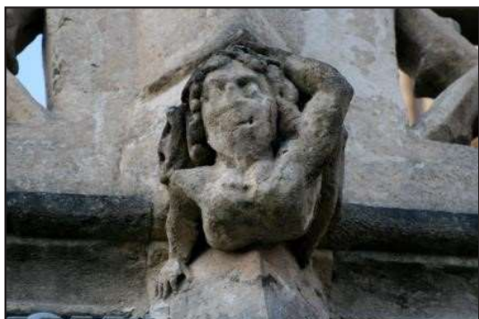
Figure 16. Degraded limestone figure on the exterior of a church in Axbridge, Somerset, England. Geomorphologists can provide insights into the characteristic weathering processes and rates on such buildings, thereby helping with the design of conservation strategies (Photo: Stephen Tooth).
