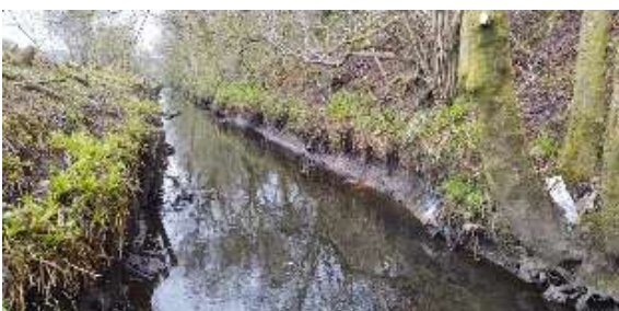
Pre-restoration condition of the Garrel Burn
