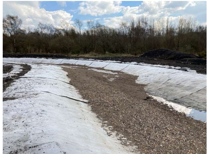
Upper reach of restored channel during construction showing clay liner.
