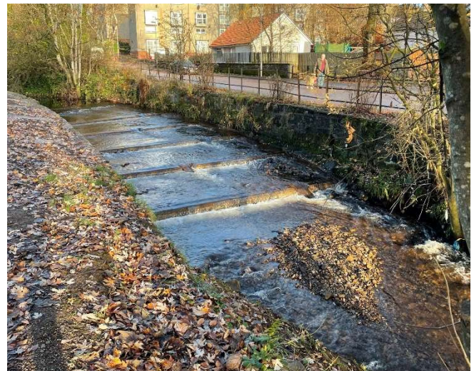
Completed pre weir to improve fish passage in November 2021.
